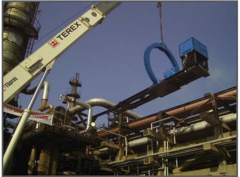
New "COBRA" line self-balancing fully electronic aerial extraction able to remove or reinstall bundle with or without your operator!
